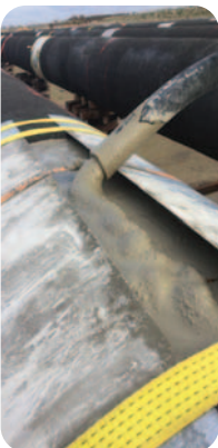
Pumping in the LA Repair Concrete
