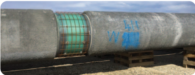
Reinforcement of the joint
